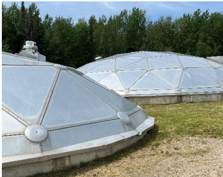
Figure 10-2: Existing CTUs at the Sioux Lookout WWTP
