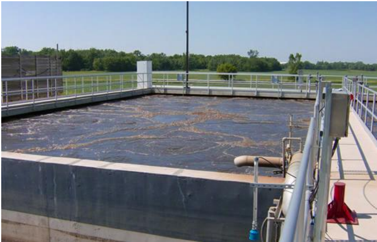
Figure 10-13: Aerobic Digester (Courtesy of APG Neuros)
