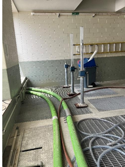
Figure 10-3: Existing Distribution Chamber
