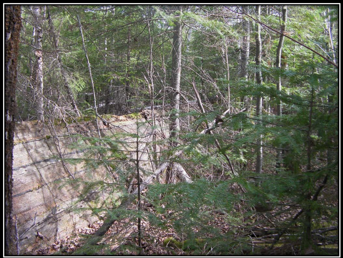
The following photos, courtesy of Bob Starratt and taken in April 2010, show the remains of scows at Second Boat Bay, Hudson.
